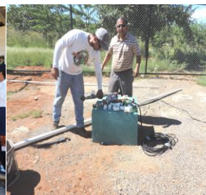
Connecting pump to well
